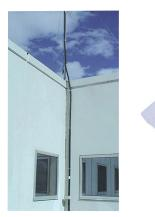
The Ericore Downconductor is easily retrofitted to existing structures. Inset: nVent ERICO Lightning Event Counter (LEC V) installed to register strikes to System 3000.
